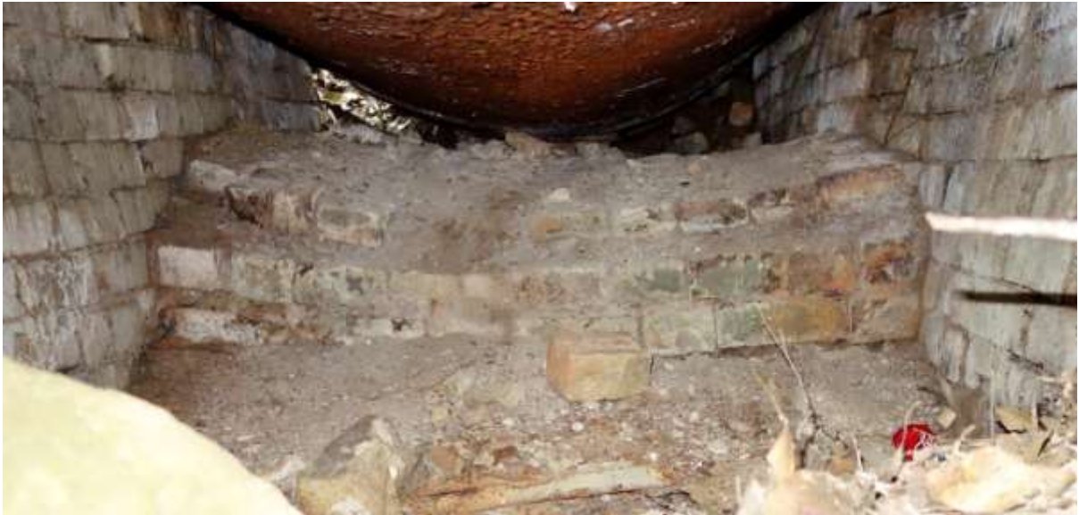
Firebox lined with Fire Bricks
