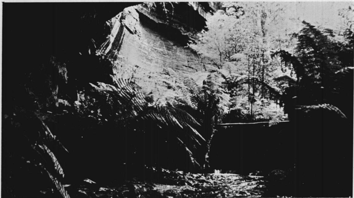
The timber bridge near the mouth of No. 2 tunnel in Penrose Gorge, 1963.
