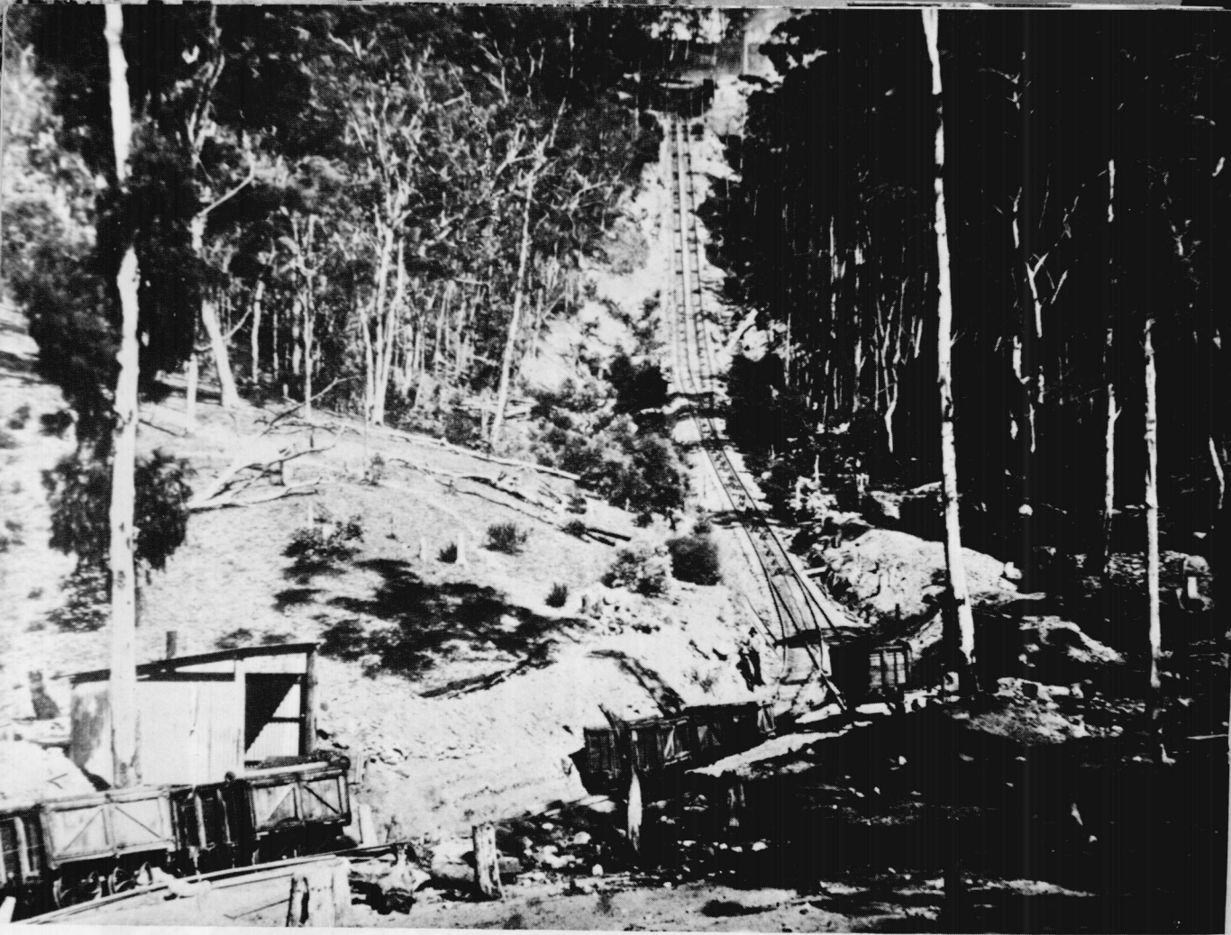
The incline to the new pit at Joadja. This was used to bring the shale to the retort house.
