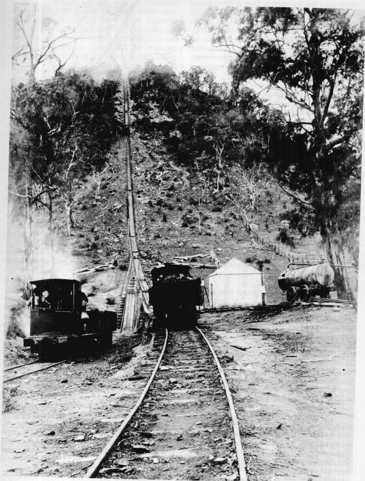
Locomotives at work at the bottom of the Joadja incline.
