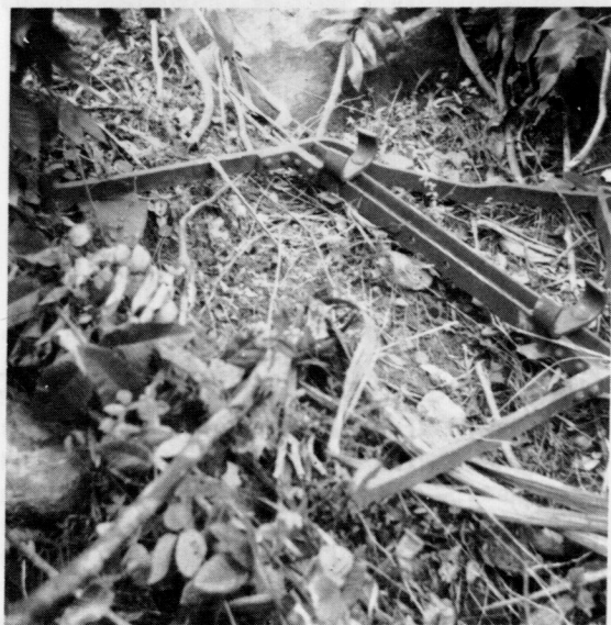
Remains of suspension bracket for buckets on Katoomba aerial cableway.
