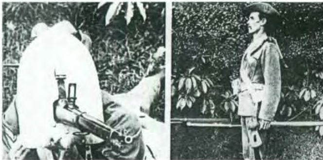
Rowe was the inventor of this ingenious but impractical shovel which also provided armoured protection of a rudimentary kind to the riflemen.
