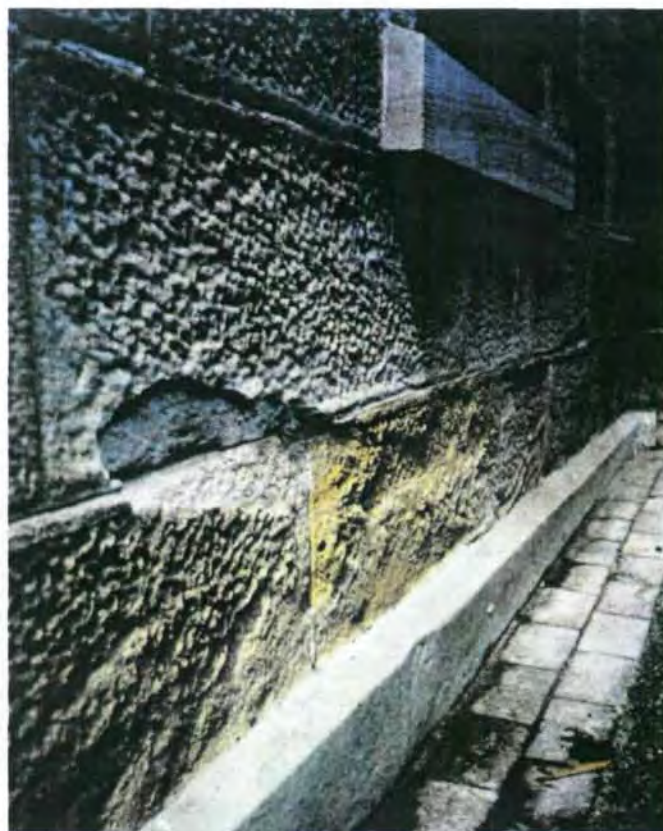
Building 13, showing exfoliated stonework caused by rising damp and exacerbated by a concrete plinth. Water permeation and termite damage also had to be rectified.
