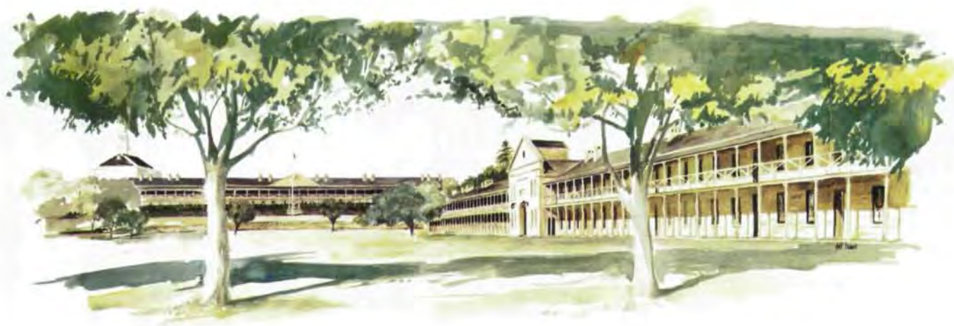
Victoria Barracks looking towards the officers' quarters. Lieutenant Colonel Barney designed the barracks to accommodate 700 British soldiers and their officers. Originally estimated to take two and a half years to build, construction time dragged on for seven years because of various delays and unforeseen problems. Total cost was about £60 000. (Painting by Jeff Isaacs)
