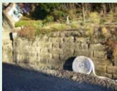
The 1866/67 sandstone abutment on the southern side of the original 1867 rail track. Note the shadow on the left that shows where the 1866-67 stone arch of the Bathurst Road bridge began.
