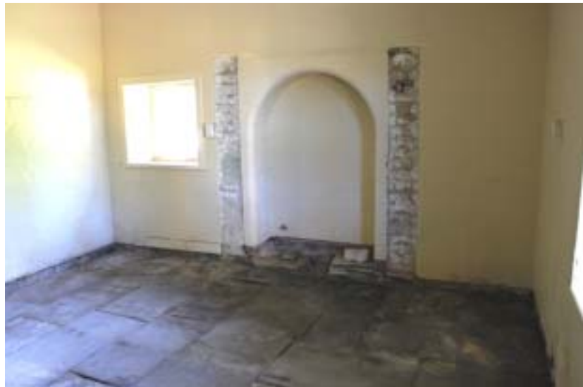
Flagstone floor and fireplace discovered during work at Eskbank House. Brick section of flooring on the right side of the fireplace
