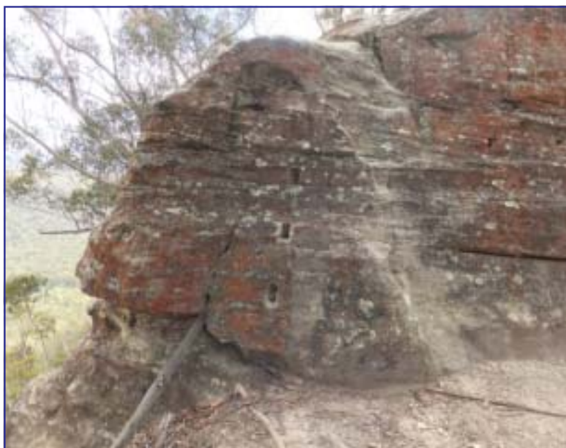
Rectangular sockets cut in the rock to receive a 3-railed fence to prevent stock from falling over a precipice along Cox's Road at Mt York
