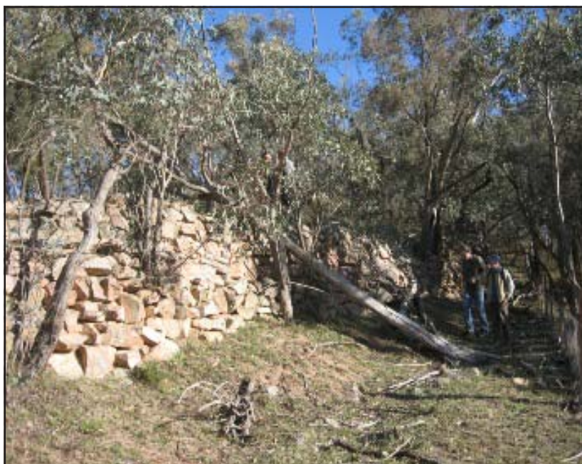
A portion of a substantial retaining wall on the zig zag of the roadway on the lower slopes of Mt Blaxland.
