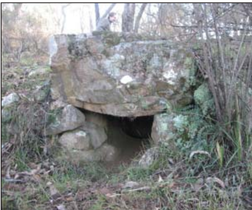
A primitive stone box culvert along the Cox's Road on the lower slopes of Mt Blaxland.
