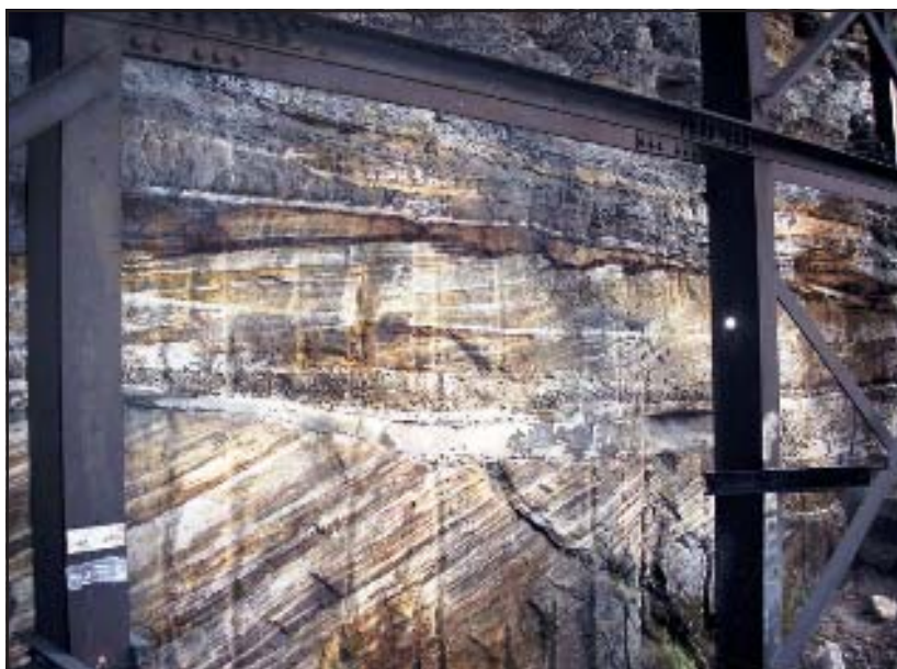
Cross bedding in sandstone on southern face of the cutting, beneath the third (steel) bridge.
