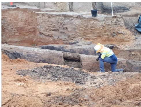
Example of brick barrel drain features
