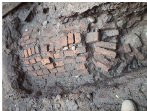
Example of brick barrel drain features
