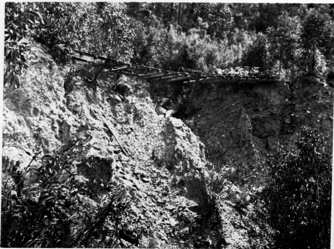
Washaways finally closed the Wolgan Valley Railway. This scour at Pass Creek typifies the damage. E.M. Stephens.
