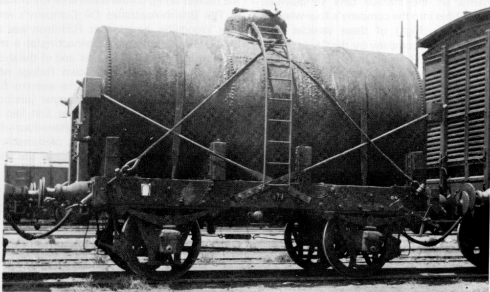
Ex-British Australian Oil Co. wooden framed oil tank wagon No. L977. The oval iron plate reads "To be returned to Murrurundi when empty." E.A. Downs.
