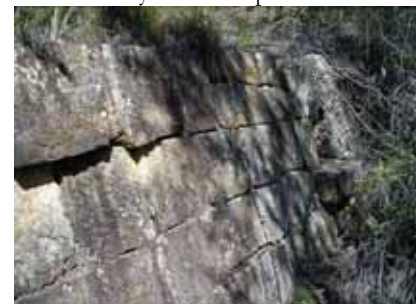
Figure 46 North face of culvert 6
