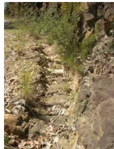
Figure 48 Drainage at base of rock cutting
