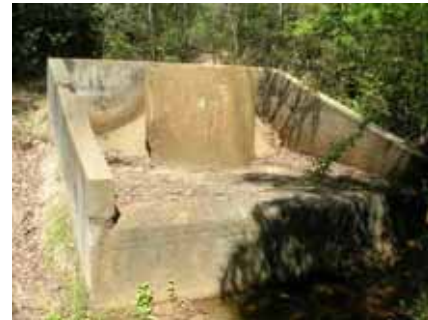
Figure 40 Energy dissipator
