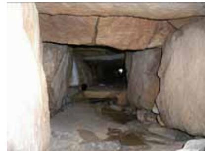
Figure 45 Structure of stone culvert below road surface
