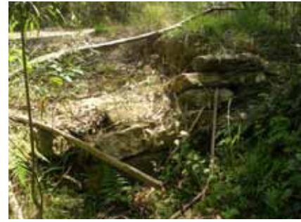
Figure 39 Retaining wall south of the culvert outlet.
