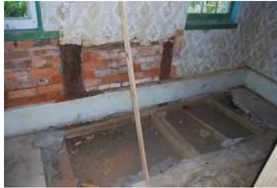
Figure 3.20 Interior photograph showing the original brick nogging construction. The timber uprights provided the structure for walls and openings and were set directly into the ground. The walls are constructed of 230mm solid brickwork (no cavity). The concrete floor and the concrete skirting were introduced in the 1930s.
