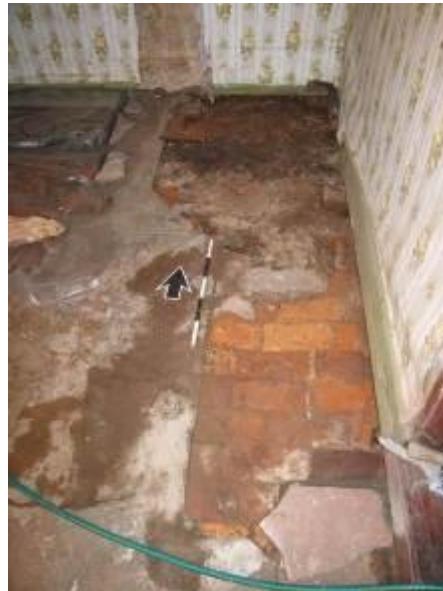
Figure 3.22 Interior photograph showing detail of the surviving sandstock brick floor in the dining room within the skillion-roofed portion to the rear of Hadley Park House.
