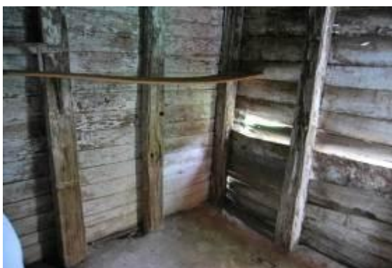
Figure 3.39 Interior photograph showing the original split timbers lined with weatherboards forming the south and east walls of the cottage.
