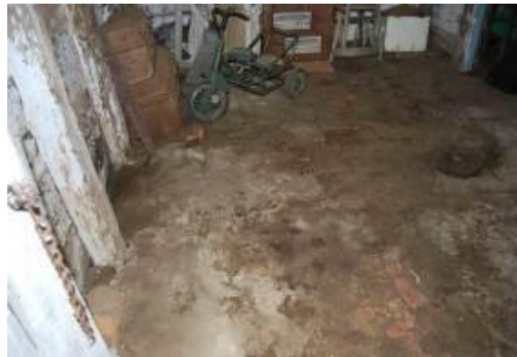
Figure 3.44 Interior detail of the Weatherboard Cottage showing the sandstock brick floor with cement covering.
