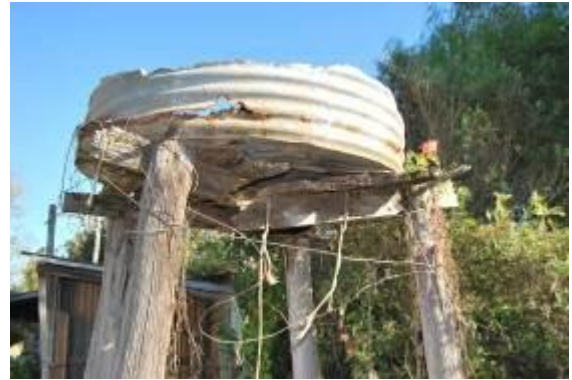
Figure 3.48 The water tank is a circular corrugated-iron tank supported by four circular bush poles, sawn timber beams and a platform consisting of sawn planks.
