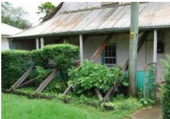
Figure 3.15 South presentation of Hadley Park House showing the privet edging along the verandah. The (temporary) props were introduced in 2008.
