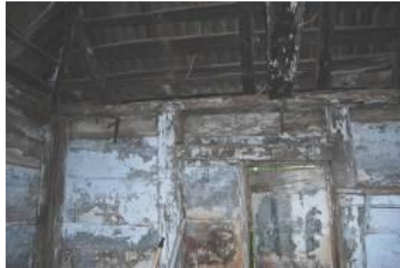
Figure 3.42 Detail of the internal wall (west elevation) showing the original structure forming the opening and original weatherboards (upper section). Note lower walling replaced with tin sheets (unknown date).
