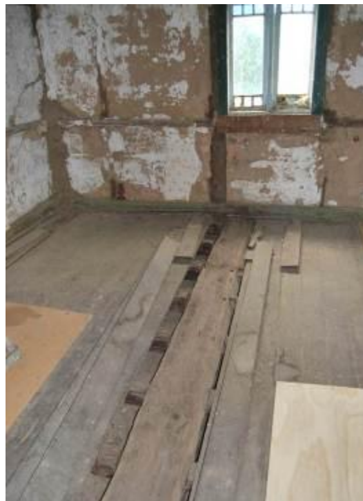
Figure 3.32 Interior view of the first floor, showing the original timber beaded skirting and chair rail and evidence of limewash finish. The timber floorboards and joists are supported on timber beams which bear onto the brickwork. Note the original opening fitted with a later window (see Figures 2.3 and 2.6).
