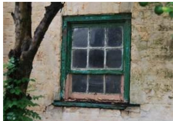
Figure 3.16 Detail of original multi-paned sash window (three small light bottom sash and six light top sash).
