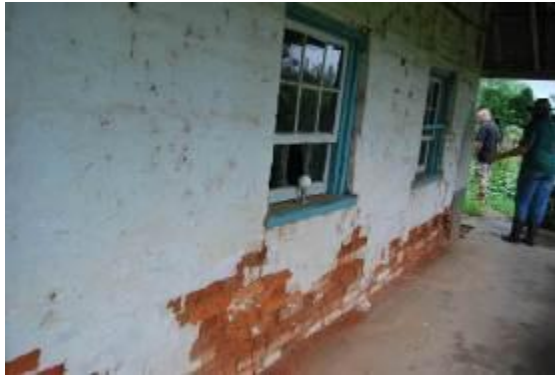
Figure 3.19 Exterior photograph showing the external brick face and limewash finish. While examples of brick nogging construction are common in the Hawkesbury Nepean area (see comparative examples in Section 3.4 below), the walls are typically plastered on the inner face, and feathered weatherboards nailed to the timber uprights on the external face. The external brick cladding at Hadley Park is uncommon.
