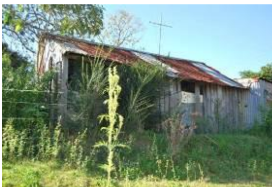
Figure 3.51 South presentation of the original portion of the former stables (or storage shed) outbuilding showing original vertical timber slab construction.
