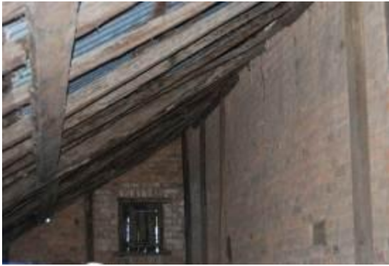
Figure 3.29 Interior photograph showing the skillion roof to the rear of Hadley Park House. Note the use of split timbers and battens for shingles.
