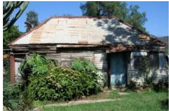
Figure 3.38 East elevation. The replacement of original weatherboards with horizontal timber boarding, corrugated-iron sheets, and the recycled panelled door and tin sheet awning illustrate the use of replacement fabric as available.
