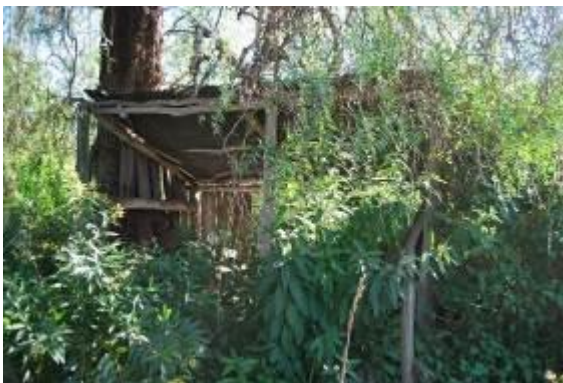
Figure 3.45 Site of the former 'wash house'. Note the use of recycled vertical timber slabs.
