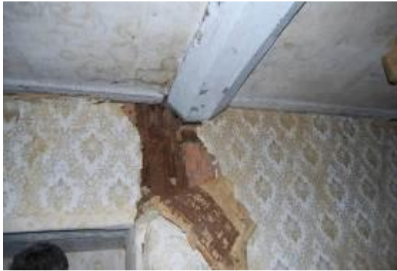
Figure 3.23 Interior photograph showing detail of the original timber post and chamfered beam at the junction, with later wallpaper covering.
