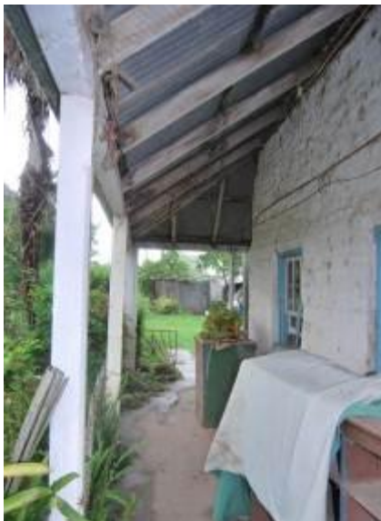
Figure 3.17 Looking south along the east verandah showing original timber chamfered posts and beams, and later rafters and battens supporting the corrugated-iron roof.
