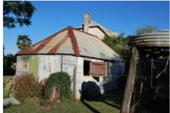
Figure 3.36 North presentation of the Weatherboard Cottage with Hadley Park House in the background. Note the original window openings fitted with tin shutters (hinged) and tin sheet walling (unknown date) on the west elevation. The elevated water tank is supported by four circular bush poles, sawn timber beams and a platform consisting of sawn planks.
