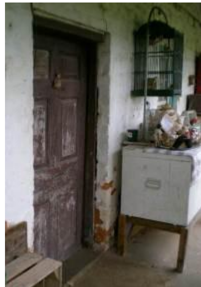
Figure 3.18 Detail of the original, typically solid, six-panelled door. Note the concrete floor (date unknown).
