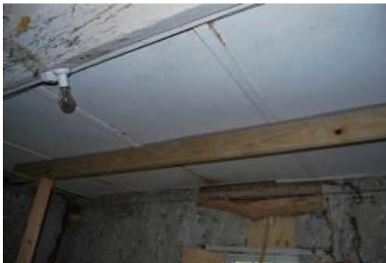
Figure 3.25 Interior photograph showing a later asbestos sheet ceiling and the recent 2008 propping.
