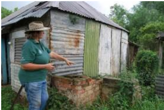
Figure 3.37 Detail of the north elevation showing the remains of the external fireplace (used for cooking) built of incombustible materials unlike the adjoining structure (typical of cottage construction). Jacqueline Flower, descendant and tenant of Hadley Park to the left.
