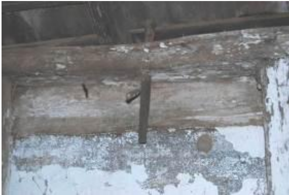
Figure 3.41 Detail of pegged (timber) joint. Note original weatherboards and replacement with tin sheeting (unknown date) below.
