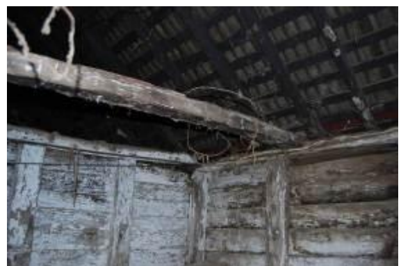
Figure 3.40 Interior photograph showing the split timbers and battens for shingles.
