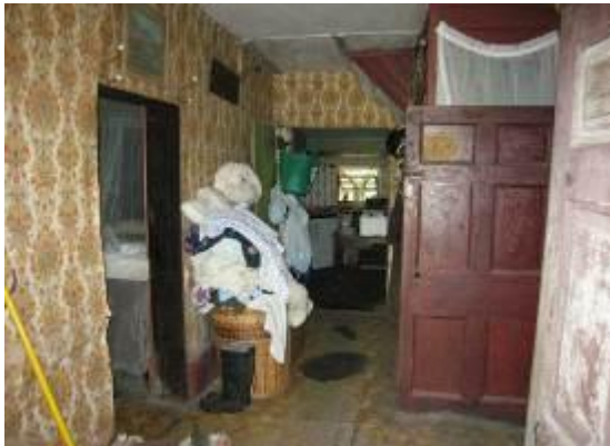
Figure 3.27 Internal view of the entrance hall (ground floor) showing the original internal solid six-panelled door and the stair leading to the first floor.
