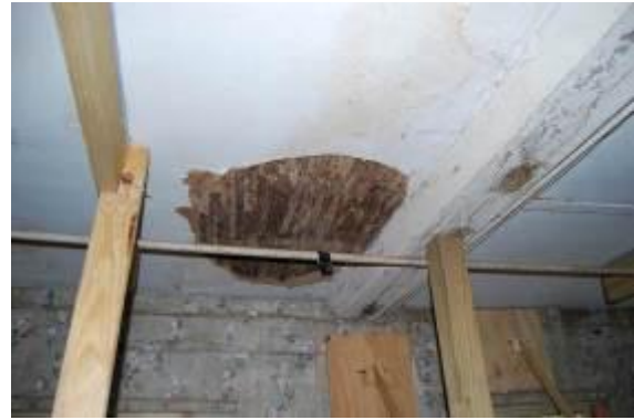
Figure 3.24 Interior photograph showing detail of the original lath and plaster ceiling and exposed timber chamfered beams. Note the (temporary) props were introduced in 2008.
