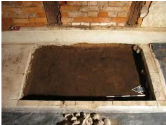
Figure 3.21 Interior photograph showing the location of the surviving timber sole plate. The timber structure has disintegrated into the soil. The floor would have been timber boards.
