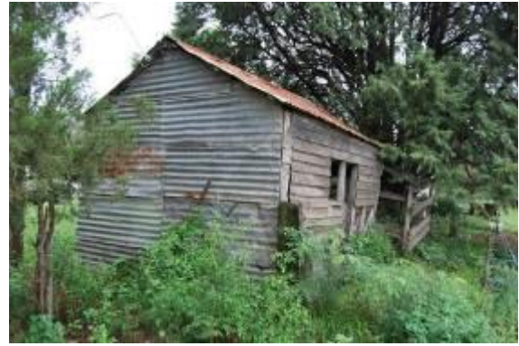
Figure 3.54 Exterior photograph of the former cream shed showing the replacement corrugated-iron sheet wall and the 1950s–1960s extension to the north.
