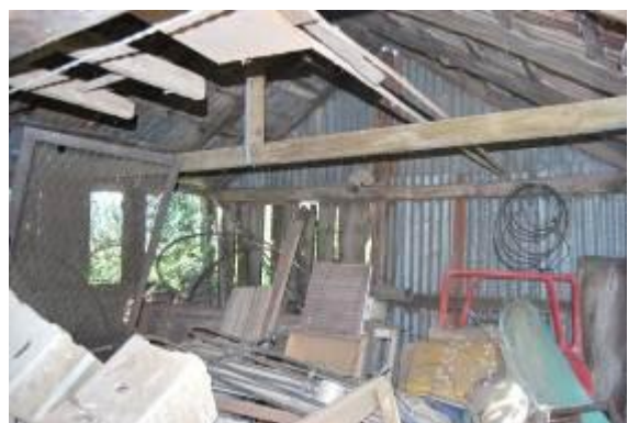
Figure 3.52 Interior view of the original portion of the former stables (or storage shed) outbuilding showing original timber slab construction and replacement with corrugated-iron sheets.
