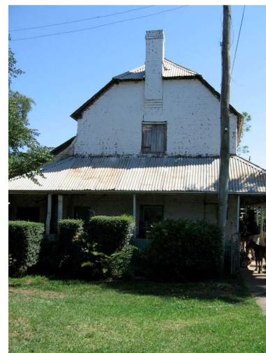
Figure 4 Hadley Park from the south.
