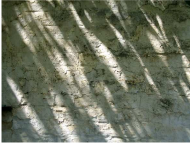
Figure 5 Hadley park masonry.
