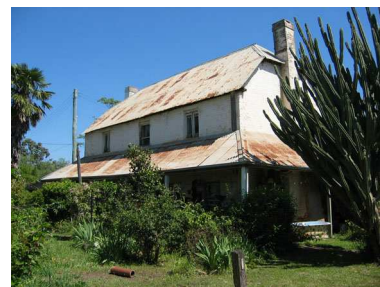
Figure 19 Hadley Park from the northeast.
