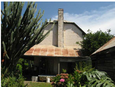
Figure 15 Garden east of timber cottage.
