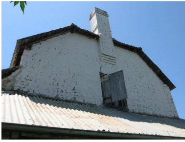
Figure 13 Hadley Park chimney.
