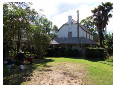
Figure 1 Hadley Park from the south
