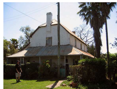
Figure 18 Hadley Park from the south.
