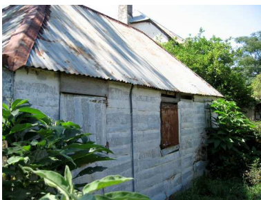
Figure 9 Timber cottage north of Hadley Park (note the metal cladding).
