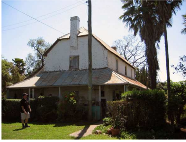
Figure 16 Hadley Park from the south.
